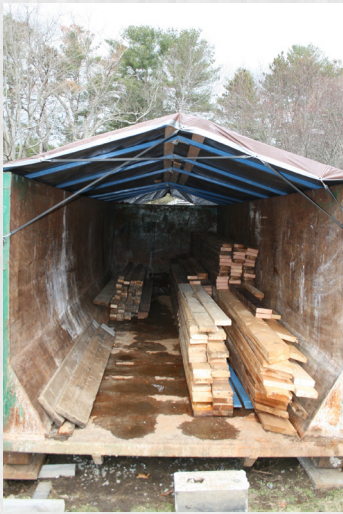
Lumber salvaged from the deconstruction of the house was collected in a 30 yard container to keep it dry, then donated to EcoBuilding Bargains.
