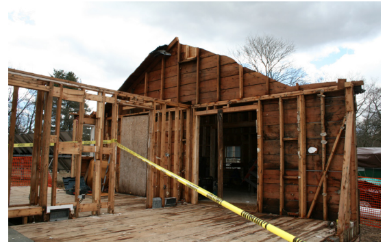
Careful deconstruction of two houses on the property ensured conservation of reusable materials.
